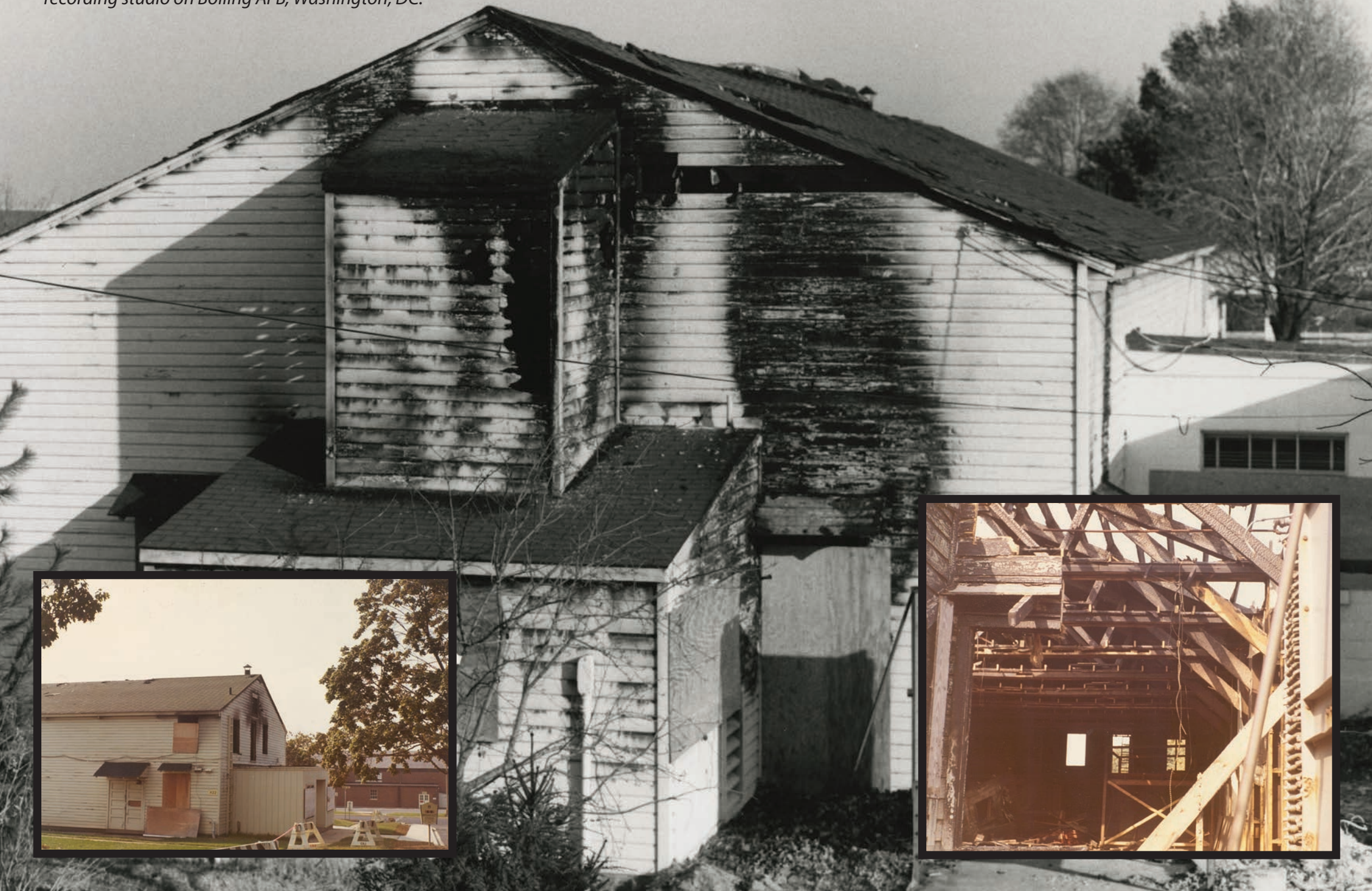
Disaster Strikes! Photos taken on August 25, 1970 following a fire the previous evening in The Band's recording studio on Bolling AFB, Washington, DC.
